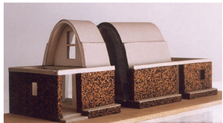
↑ HUDCO Housing: The competition was to design post-disaster housing, selecting a village in Kutch. Research revealed that much havoc resulted due to failure of walls because of missing key stones in the masonry. A cross-sectional model showing the material layers to provide strength to the roofs making innovative use of local resources was developed.
