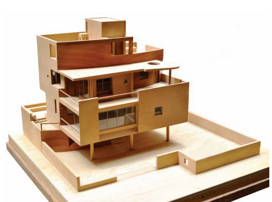
↑ Bindiben House, Bharuch: The entire house is raised on a hollow plinth to access views of river Narmada flowing near the site. Private spaces such as bedrooms are placed behind the curved wall. Living and dining areas are pulled out from the curved wall, which with large openings, frames views on the river side.
